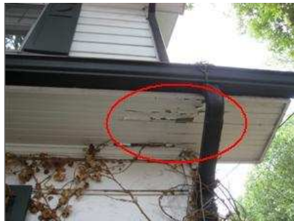
2.5 Picture 3 Front (right of main entry)
