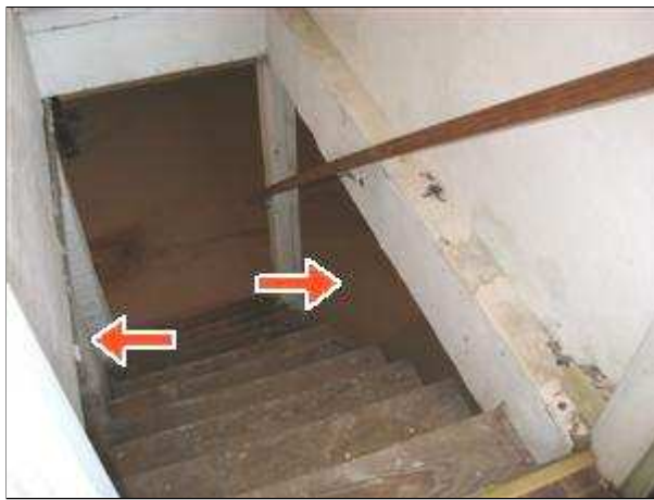
3.3 Picture 1 basement stairs
