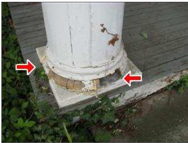
2.3 Picture 1 Front Porch
