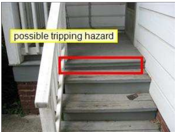
2.3 Picture 2 Rear Porch
